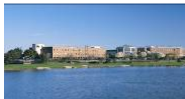
Delnor Hospital Illinois
